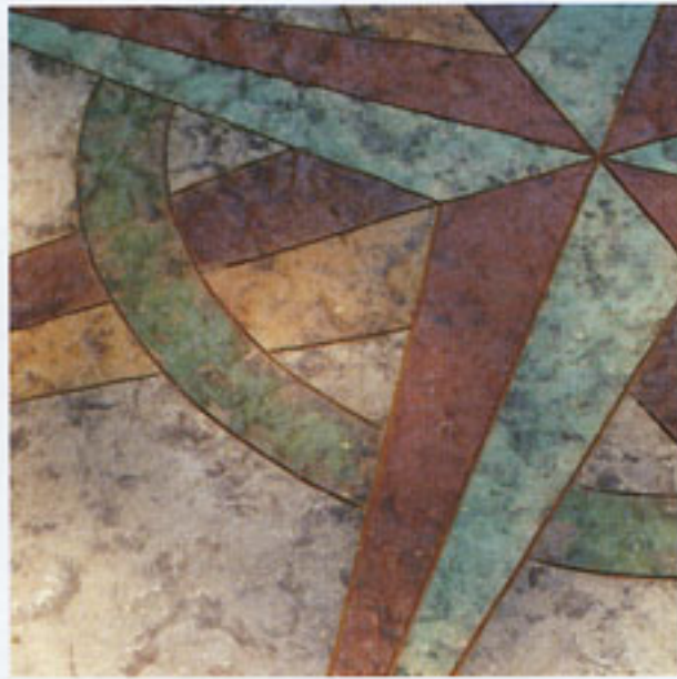
Durability and exciting effects can be achieved when LITHOCHROME® Chemstain™ Classic or LITHOCHROME® Tintura™ Stain is applied over textured LITHOCHROME® Color Hardener.
